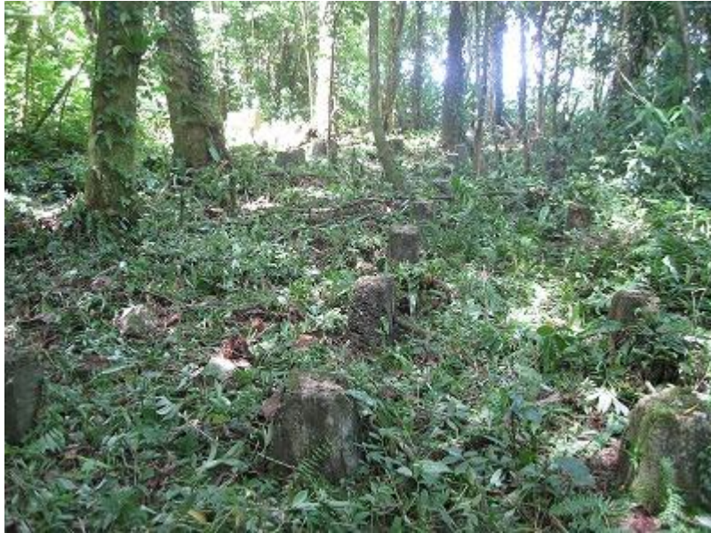
Figure 77. Concrete post of a barrack.
