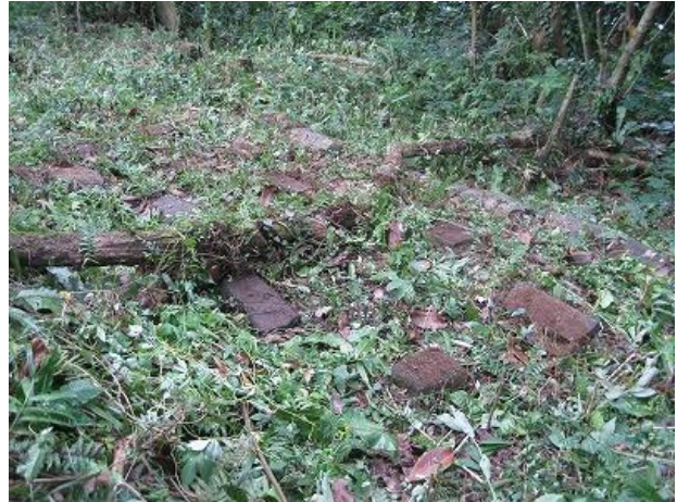
Figure 71. The southern foundation.
