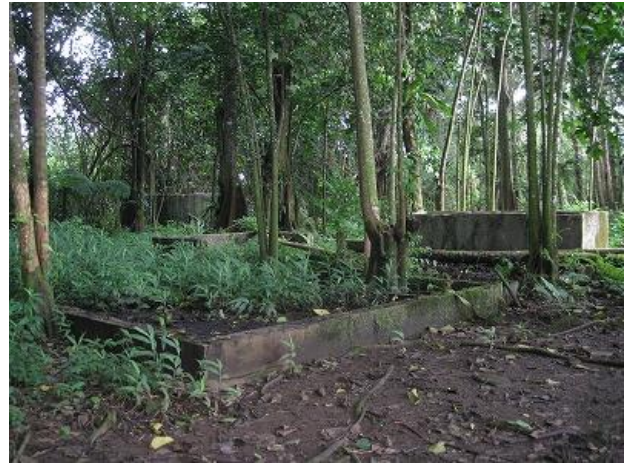
Figure 50. Kitchen-mess hall foundation.
