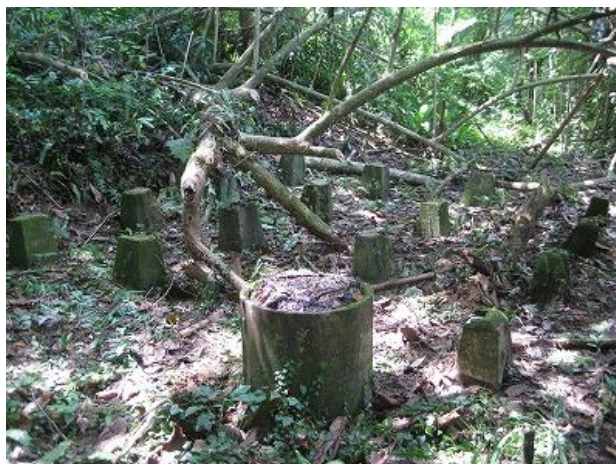
Figure 65. Concrete foundation posts.
